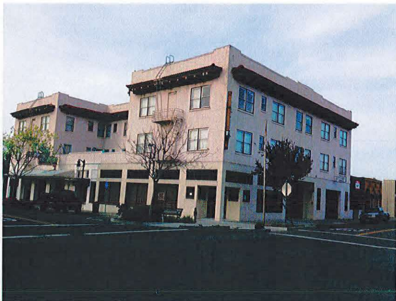
Rio Vista Hotel, purchased May 2013, renovation is beginning.
